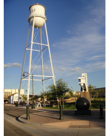
Gilbert. Water Tower
